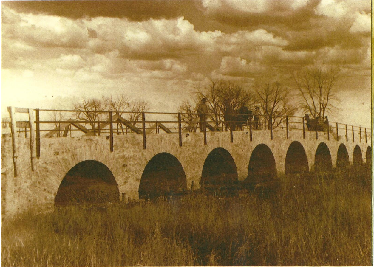
Alphonse Halter on his newly built bridge in 1901
